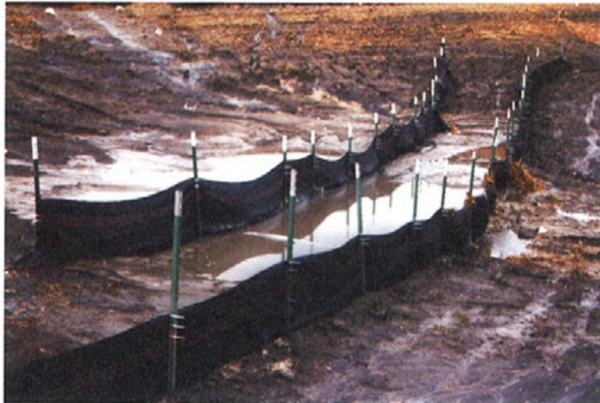
A new fence is often a better solution than cleaning an old fence.
