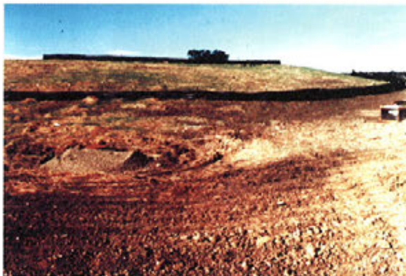
Fence at head of slope decreases volume of water and erosion potential.
