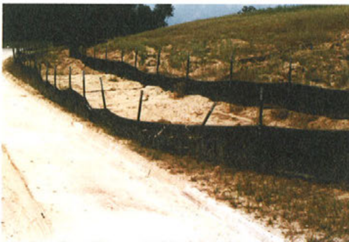
Steel posts will hold the weight.
