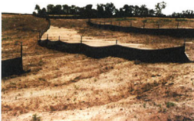
Proper Installation. One 100 ft. run of silt fence could hold 50 tons of sediment!
