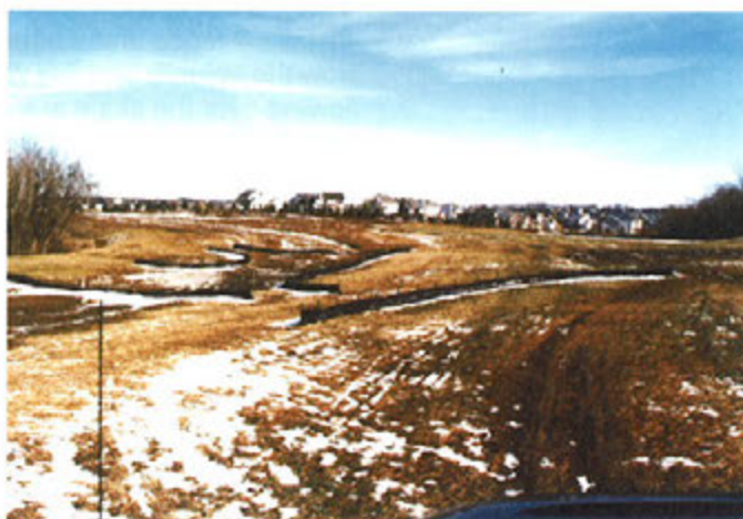
Multiple runs diffuse the volume of sediment laden water.
