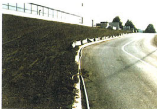
poor placement - funnels water to end
