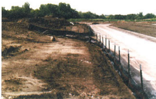
A hook is required on most silt fence runs to pond water
