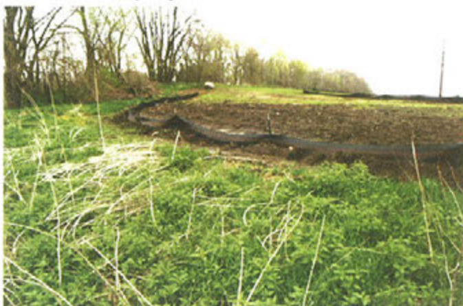
Improperly maintained silt fence
