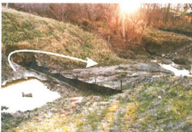
Poor installation can cause severe erosion around the end
