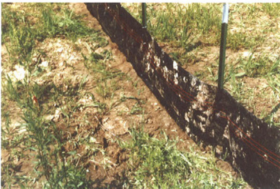
Compact Soil Prevents Piping and Washouts
