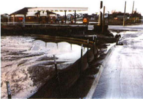
Protect stormwater inlets before sediment gets onto streets.
