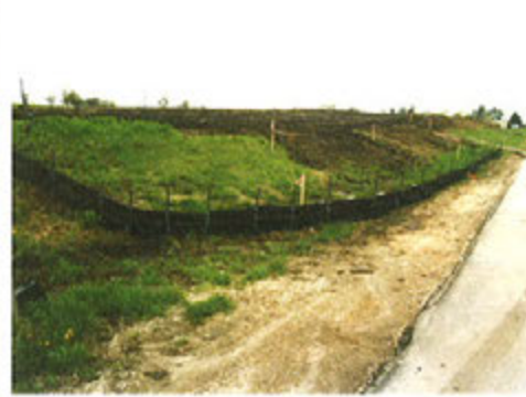
Silt fence turned up to create a dam
