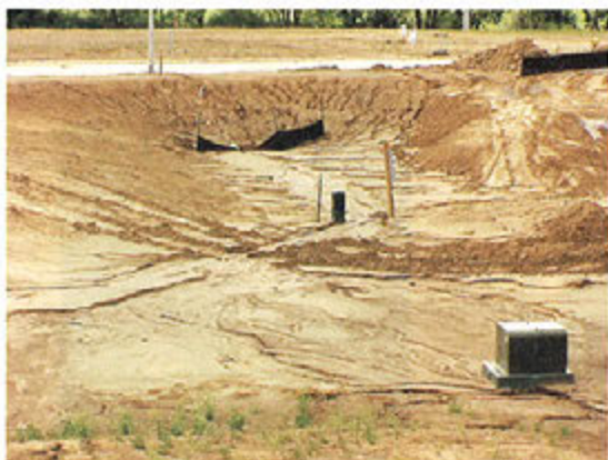
One control at outlet is not adequate
