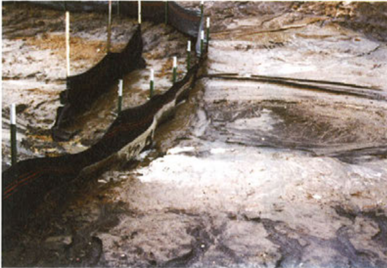
No Compaction = Under-Cutting
